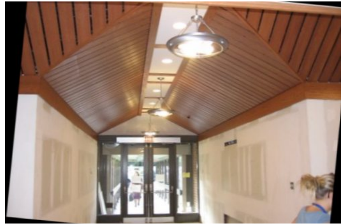
The New Ceiling Under Construction photo by K. Katzell
